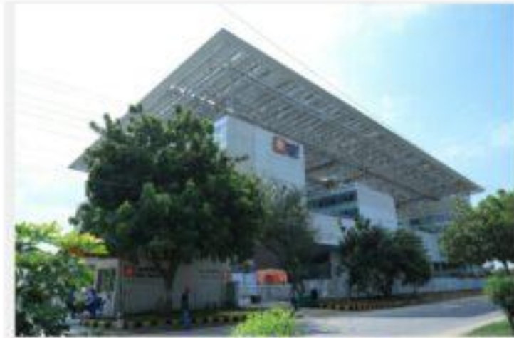
REC Limited HQ building
