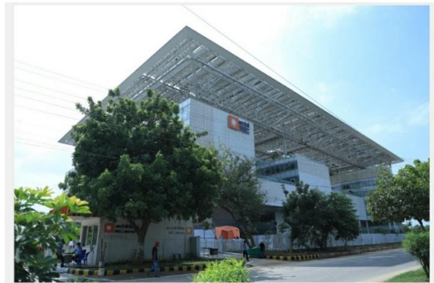
REC Limited HQ building
