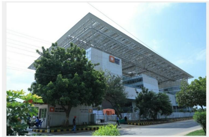
REC Limited HQ building
