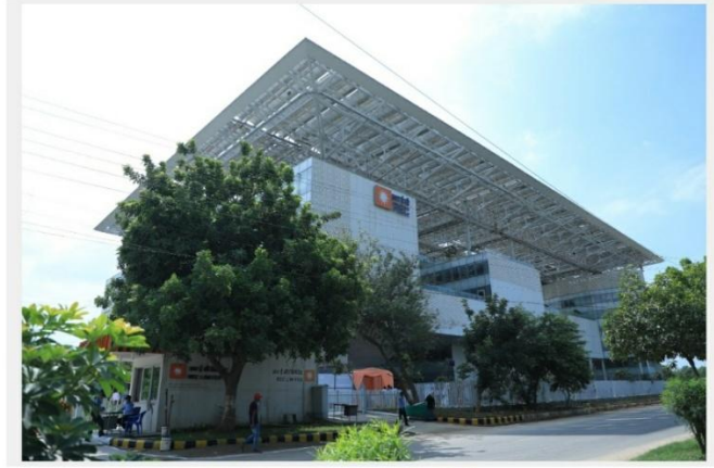
REC Limited HQ building
