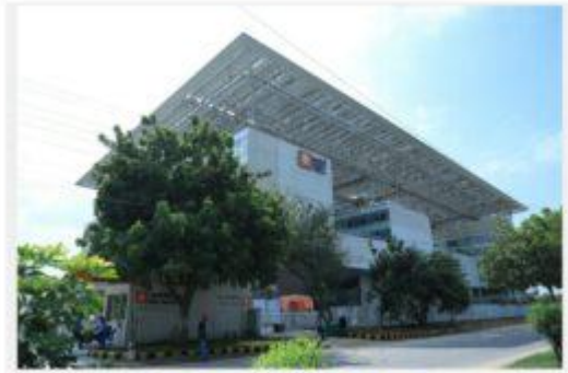
REC Limited HQ building
