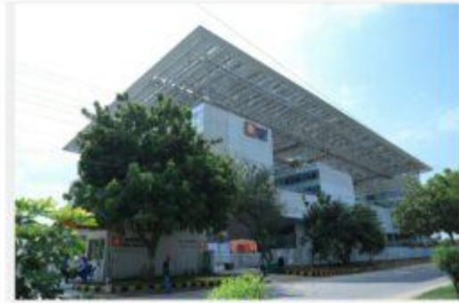
REC Limited HQ building
