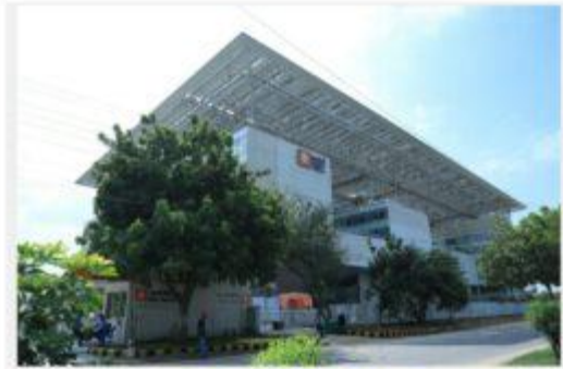
REC Limited HQ building
